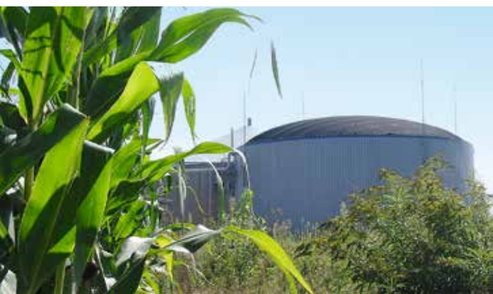
Biogasanlage in Neuried
